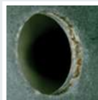
6 months (galvanised steel) 30-40% red rust 60% white rust
