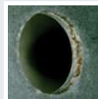
6 months (galvanised steel) 30-40% red rust 60% white rust
